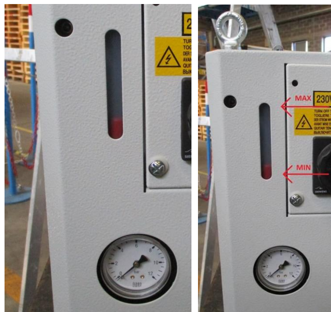
Picture 13/14 – tank top up
