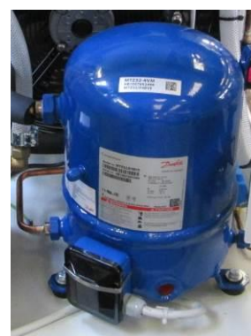
Picture 17 – Compressor placement for nBoxX 3.5 , nBoxX 5.0 , nBoxX 6.5
