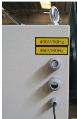
Picture 10 – Electrical connections
