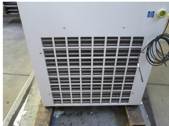
Picture 20 – Condenser external surface for nBoxX 3.5 , nBoxX 5.0 , nBoxX 6.5
