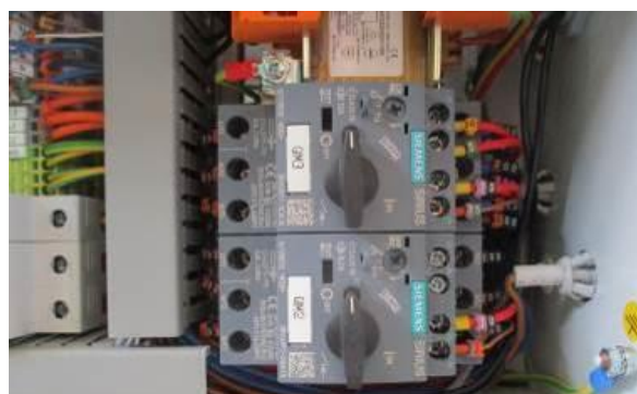
Picture 11 – pump breaker On
