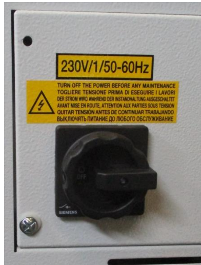
Picture 12 – Main switch ON
