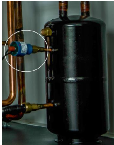
Figure 3 High Pressure Limiter Location
